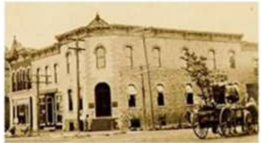
1882 – 1892 (Lyons Bldg/Burlingame Bank)
